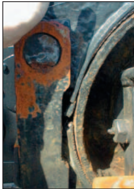
Maintenance, or lack thereof, plays an important role in the operation of deck machinery.
